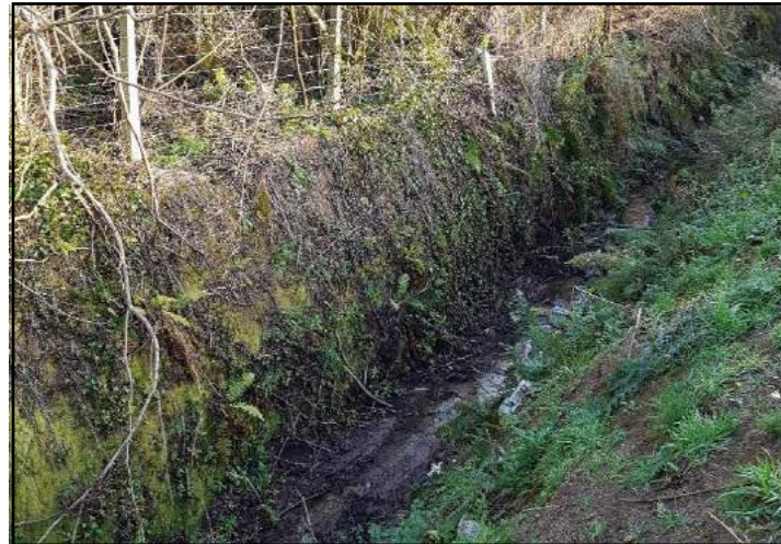
Plate 10: Section of the drainage ditch (FW4) at the site.
